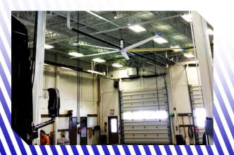
The Altra-Air Sailfin variable pitch, modulated trailingedge airfoil removes the inefficiencies created by differentiating rotational HVLS Fan speeds.
